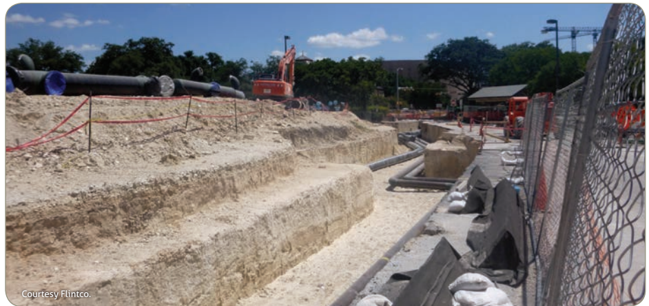
View of the new thermal distribution trench excavated within solid limestone subgrade. The trench will contain both hot and chilled-water piping.
